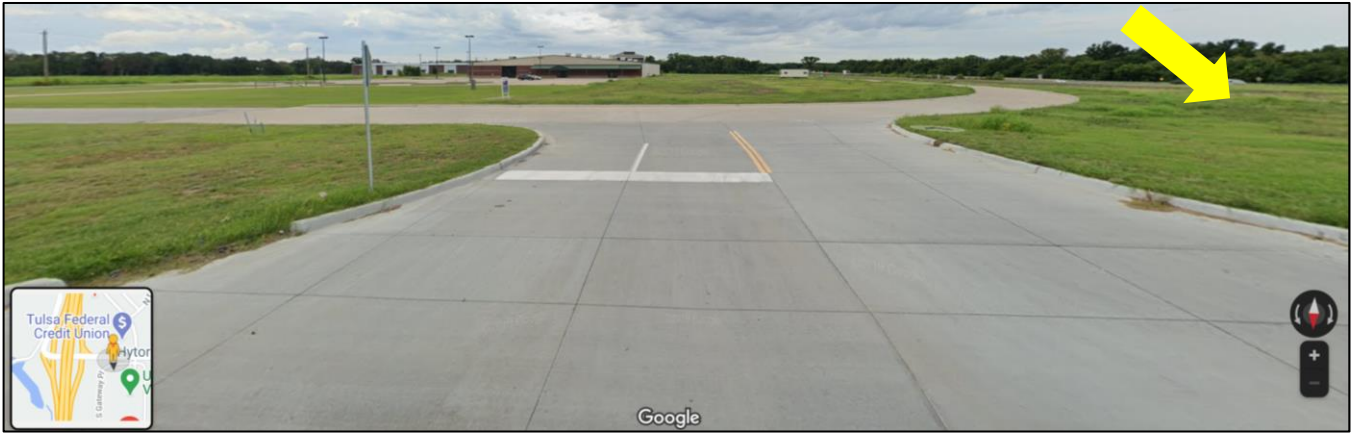
Figure 4: Google Map South view from Main Street & N. Douglas Street
