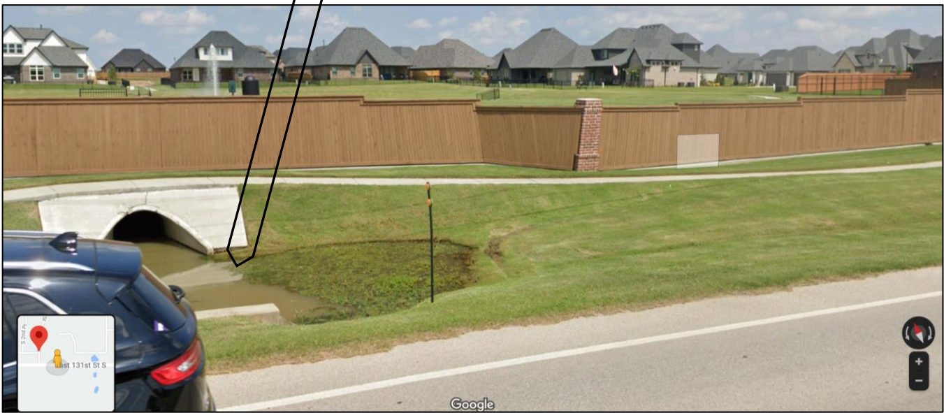
Figure 6: Google Map | Street View of Drainage Structure | 131st Street
